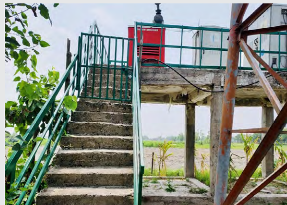
Infrastructure elevated to combat flood impact
